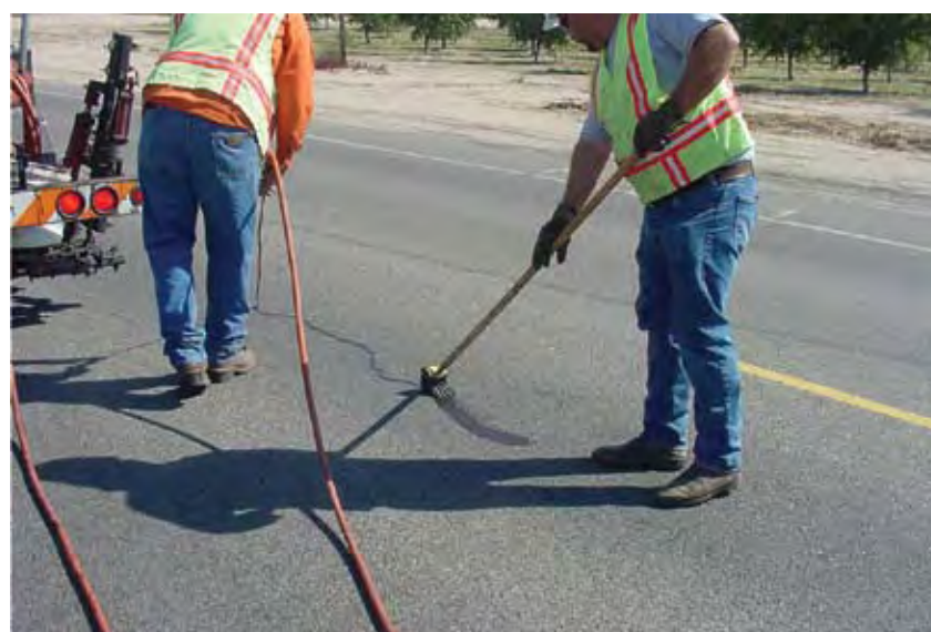
Crack Sealing
